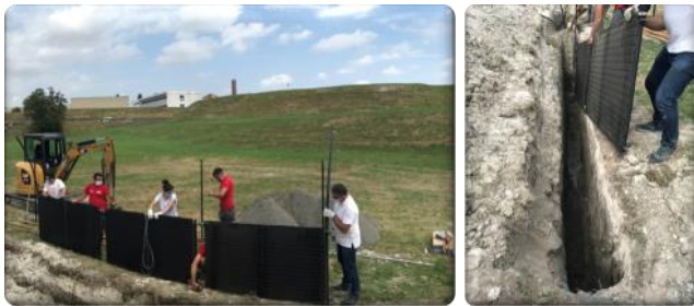
Flat Panel GHX trench installation
