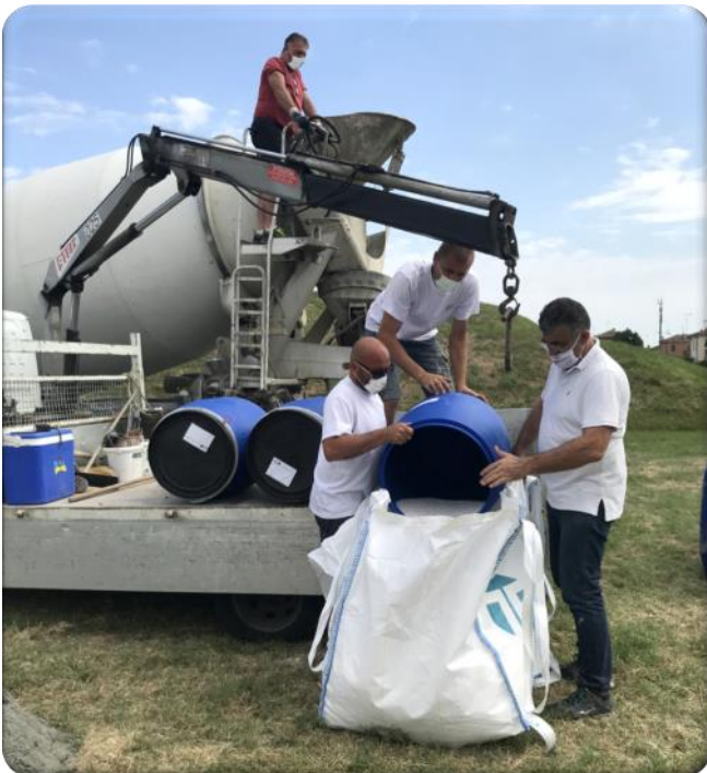
Paraffin granule PCM mixed with sand
